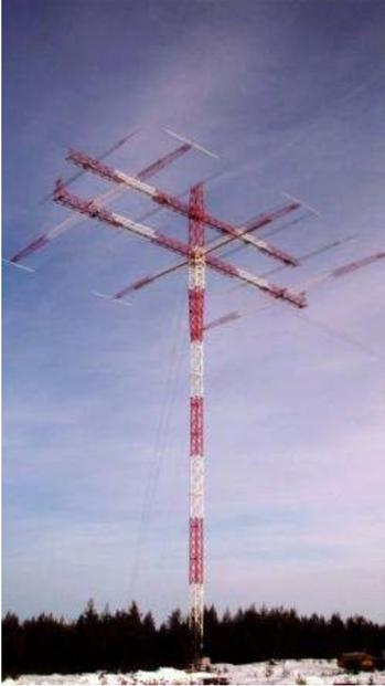
It's well known that the bigger and higher the antenna, the better results you'll get. The new 3-element 160m antenna at **OH8X** must be about as big as you can get. Look out for a strong signal from them during 2009. The new antenna for the 160m Amateur Radio band was completed just in time for Christmas on 24th December after OH8SR and OH6RM had spent three weeks installing it. The Arcala Extremes station OH8X is located at Arkala 65.18N, 26.24E.
